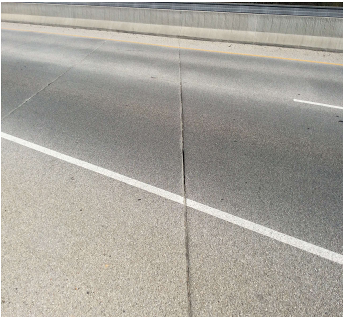
PHOTO 1 Description Saw joint sealant deterioration.
